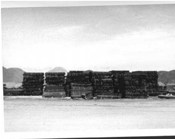
Marston Mat, more properly called pierced steel planking (PSP), is standardized, perforated steel matting material used for temporary runways and driving surfaces. Here, stockpiled along Route 19.
